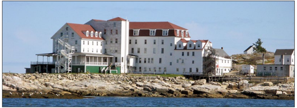
The new red roof on the Oceanic Hotel was paid for using your contributions to the Shining the Star campaign. Thank you!
